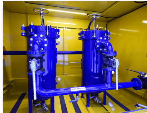
Welded manifolds reduce the potential leak points and pipe labels make operations simple
