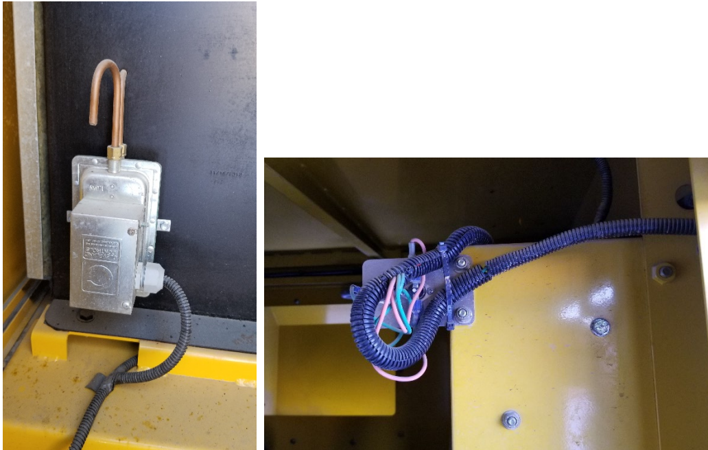
Figure 7. Burner and Safety Controls
