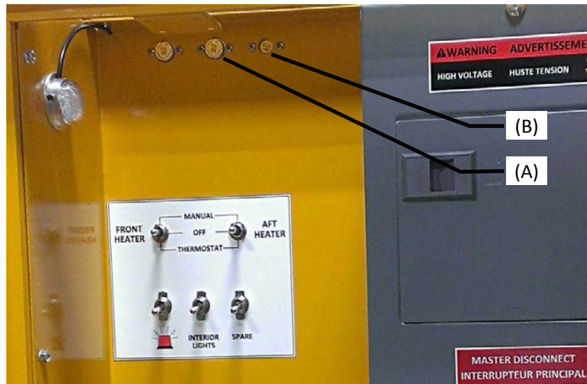
Figure 4. Enclosure over-temp thermostats (A) and enclosure cooling fan thermostat (B)
